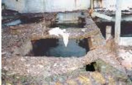
Gambar 2.5 Korosi Merata (*uniform corrosion*)
