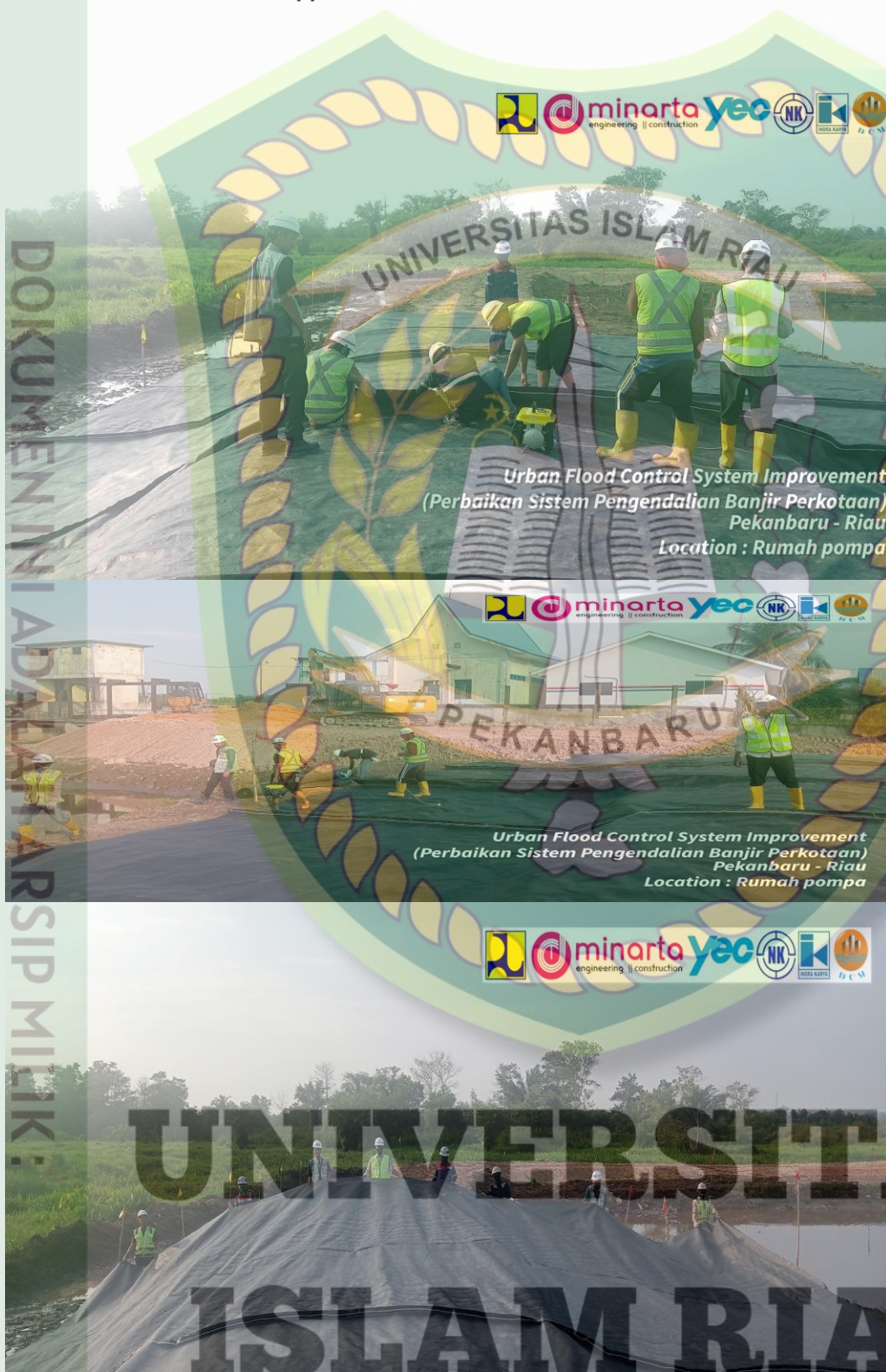
Figure 7.21 Woven Geotextile Installation at (UFCSI)
