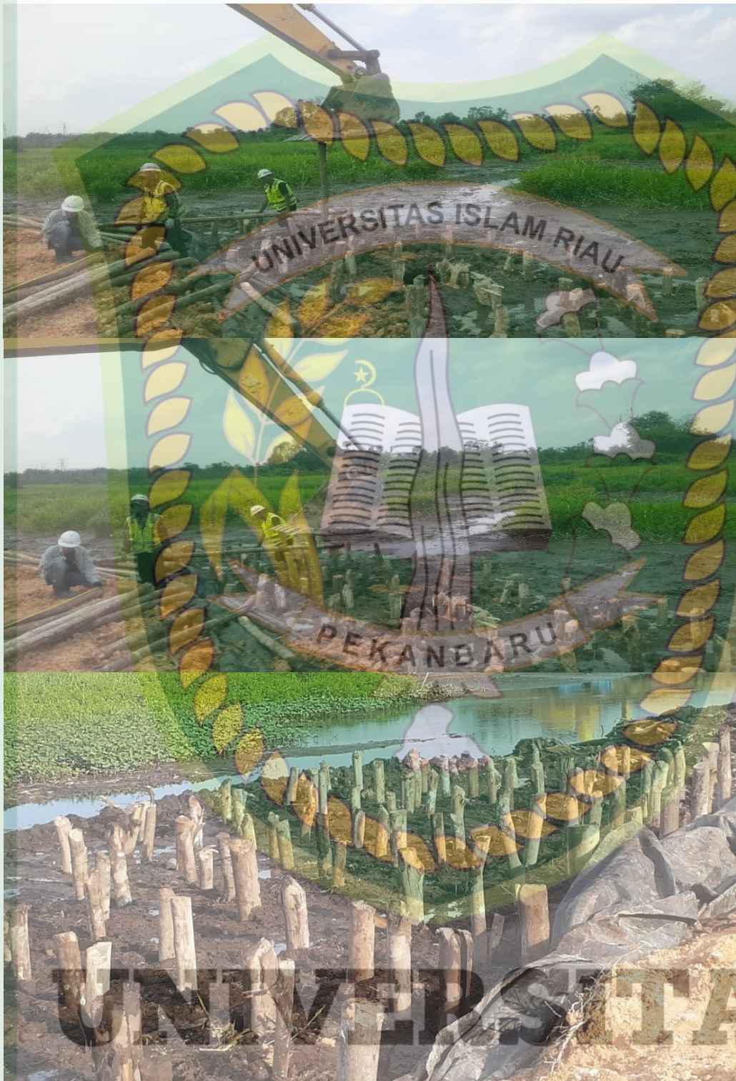
Figure 7.20 Cerucuk wood installation at UFCSI Jl Nelayan Rumbai Pekanbaru Indonesia
