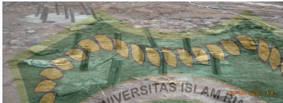
Figure 3.3 Micro piles soil reinforcement (Sun, 2014).
