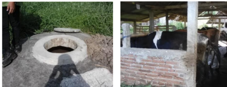
Fig 12. Tank Installation of Biogas & Communal Sheds
