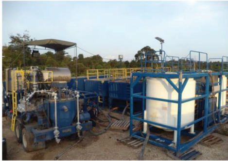
FIGURE 3a. Surface facility for chemical storage (Zulfikar et al., 2014).
