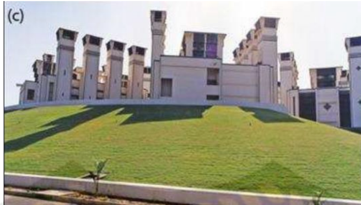
Gambar 2.11 Gedung Pusat Penelitian Torrent di Ahmedabad di India Sumber : (Hughes, Chaudhry, & Ghani, 2011)
