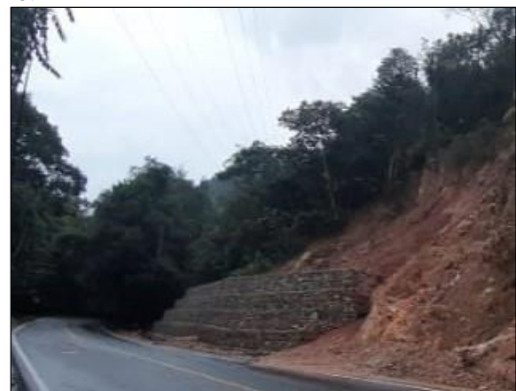
Fig. 23. Landslide Mitigation with Retaining Rock Embankments
