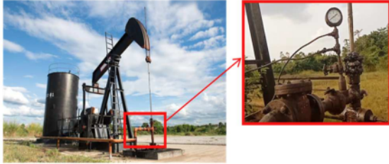
Fig. 1. Illustrated of oil well on the field and parts to monitor
