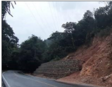
Fig. 23. Landslide Mitigation with Retaining Rock Embankments
