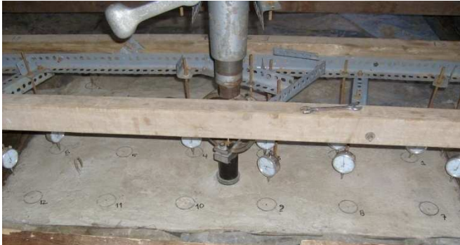
Fig. 5. Photograph of center loading test on nailed-slab with two rows of piles.
