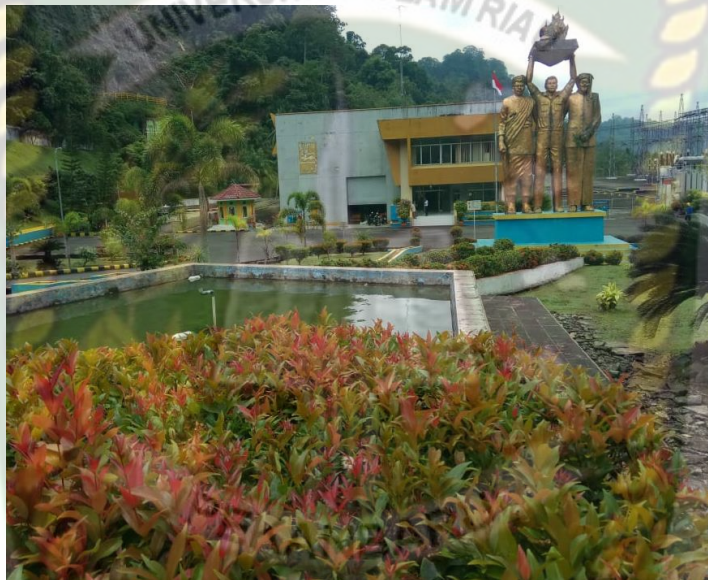
Gambar 3.1 Power House PLTA Maninjau
