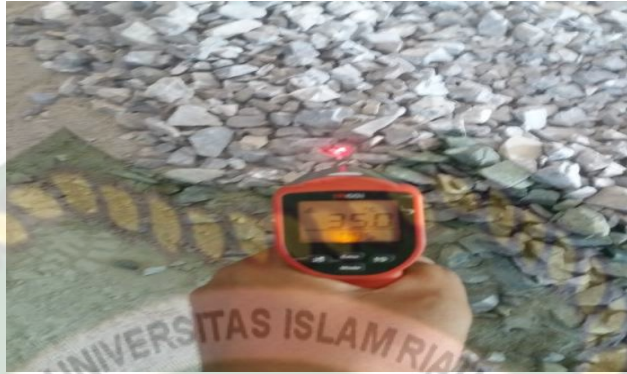
Gambar 4.7 Pengecekan suhu agregat kasar 35^{\circ}\text{C}\pm 1 (Dokumentasi, 2020)
