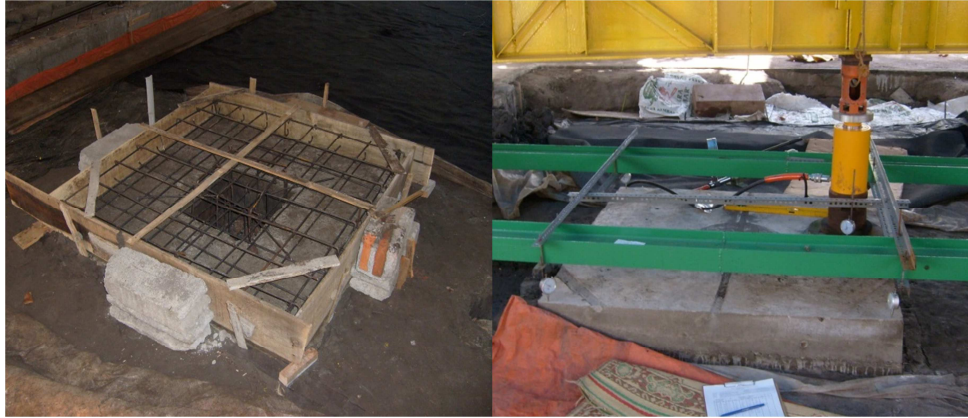
a) Slab reinforcement
