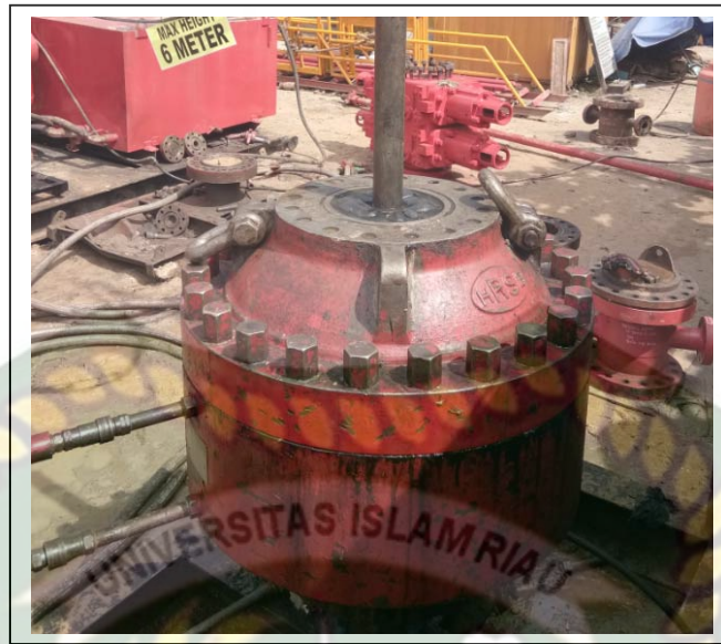
Gambar 2.6 Pengetesan well bore (ACS data)
