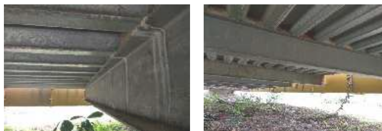
Gambar 5.5 Kondisi Cross Beam .
