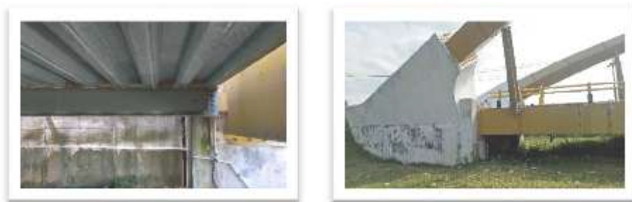
Gambar 5.1 Kondisi lapangan Abutment .
