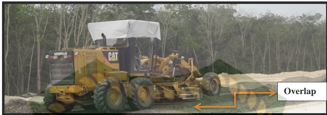
Gambar 5.13 Overlap pada saat penghamparan agregat
